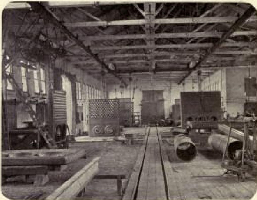
INTERIOR VIEW OF ASSEMBLING SHOP.
