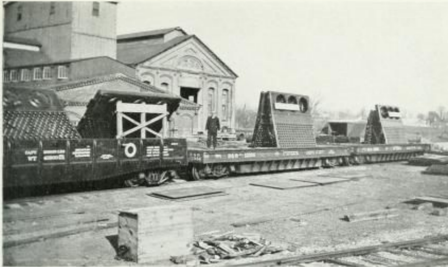
Typical loading of large Edge Moor headers
