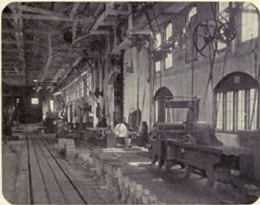
INTERIOR VIEW OF MACHINE SHOP.
