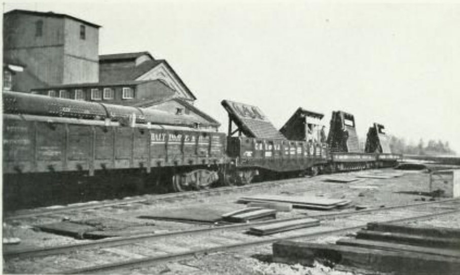
Shipment of three 600 horsepower boilers leaving the works
