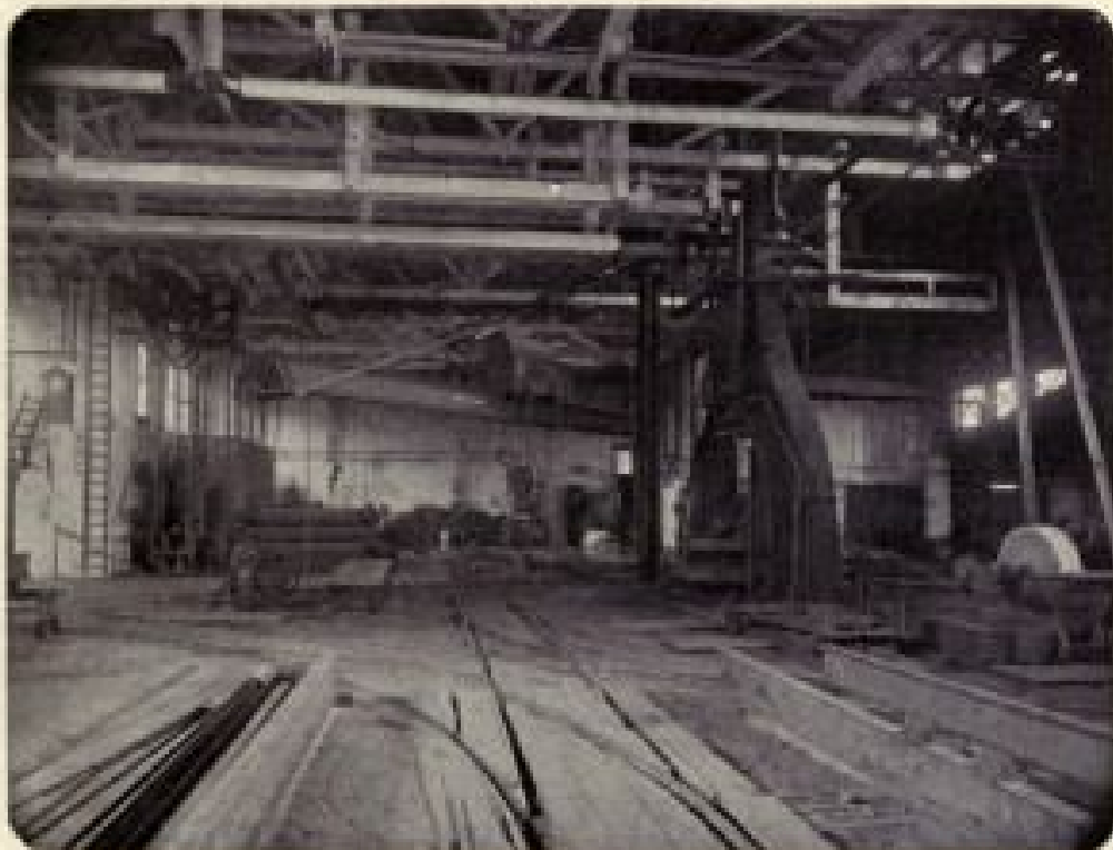
INTERIOR VIEW OF FORGING AND RIVETING SHOP.
